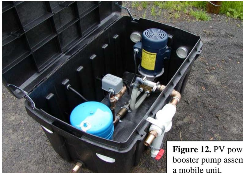
**Figure 12.** PV powered booster pump assembly in a mobile unit.
