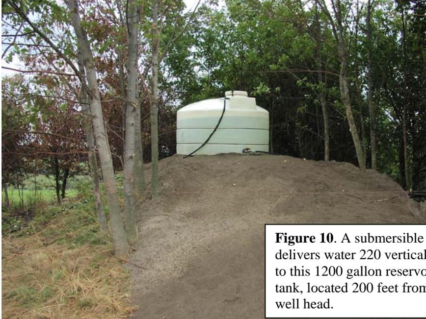
**Figure 10.** A submersible pump delivers water 220 vertical feet to this 1200 gallon reservoir tank, located 200 feet from the well head.
