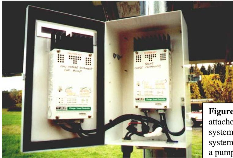
**Figure 9.** A charge controller attached to the array for a system with batteries. For a system without batteries, only a pump controller would be installed.
